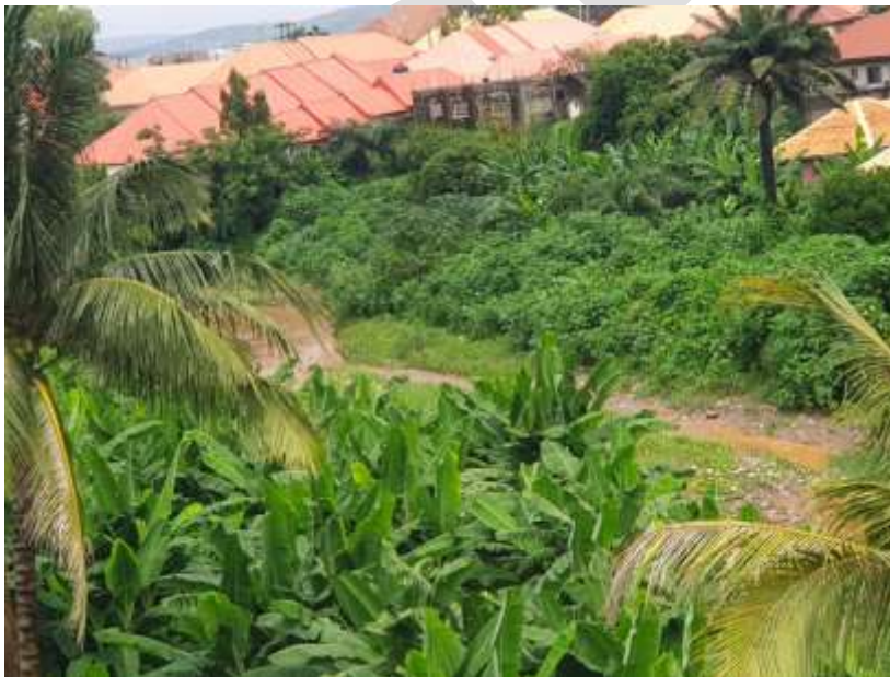
Figure 4: Path of Water Discharge on the Site
